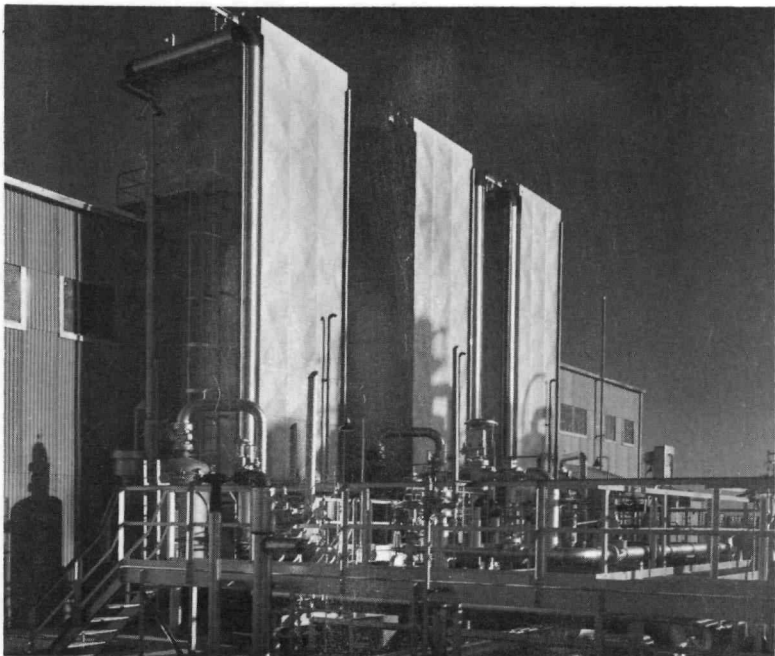
Figure 1 A U. S. Bureau of Mines helium plant in Keyes, Oklahoma, with the "cold boxes", or refrigerating units, in the foreground.
